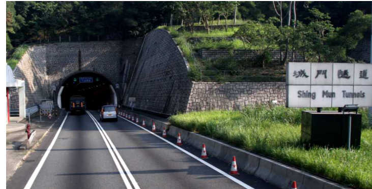
Shing Mun Tunnels / Hong Kong
