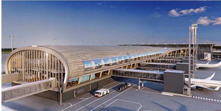
OSLO Airport / Norway
